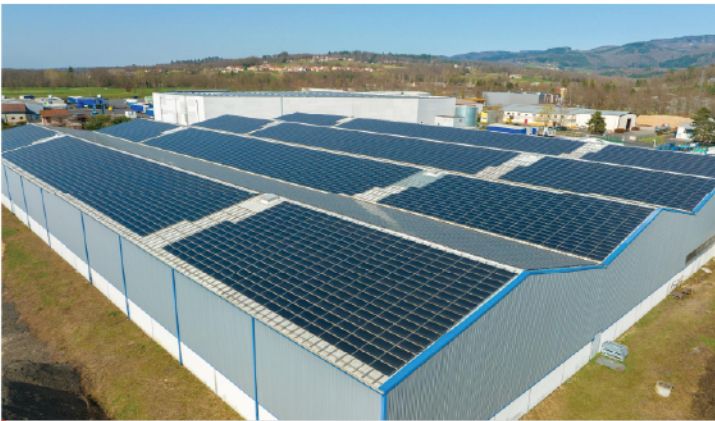
SOLAR ROOFTOP - INDUSTRIAL/COMMERCIAL
